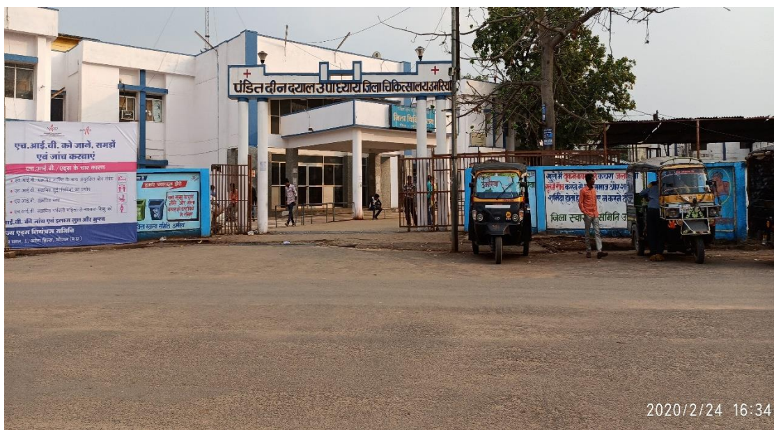
Figure 11: PDU District Hospital Umaria
